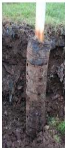
Vertical Gas Venting Pipe installed on Pipe Connection Pit
