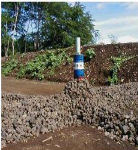
Vertical Gas Venting Pipe installed on Pipe Connection Pit
