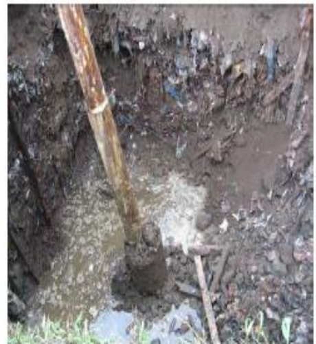
Vertical Gas Venting Pipe installed on Pipe Connection Pit
