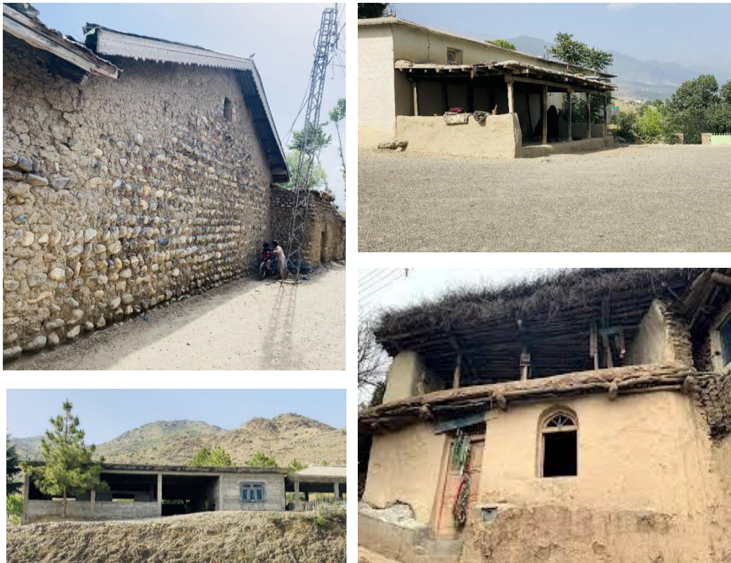
Figure 4-1: Existing Condition of Residential Buildings
