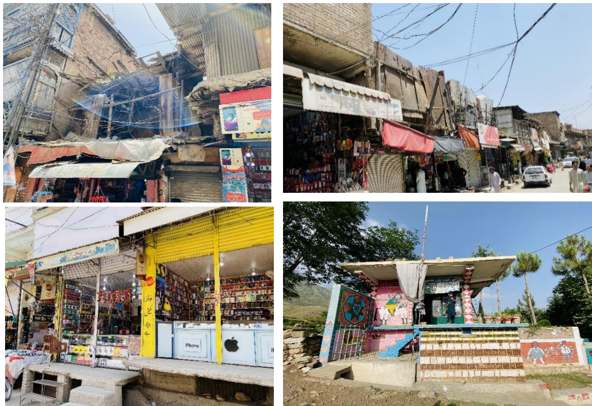
Figure 4-3: Existing Condition of Commercial Area
